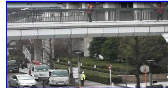
(8) On pedestrian bridge
