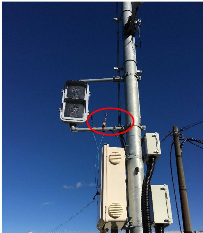
**Fig 3.4.1-6 Signal Post B (radio antenna indicated by the red circle)**
