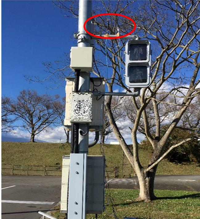
**Fig. 3.4.1-5 Signal Post A (radio antenna indicated by the red circle)**
