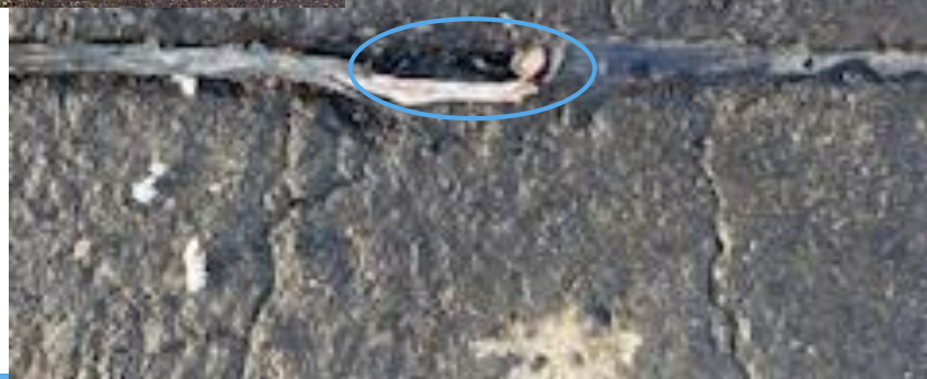
Disconnected ⇒ due to the effects of snow removal work, etc.
