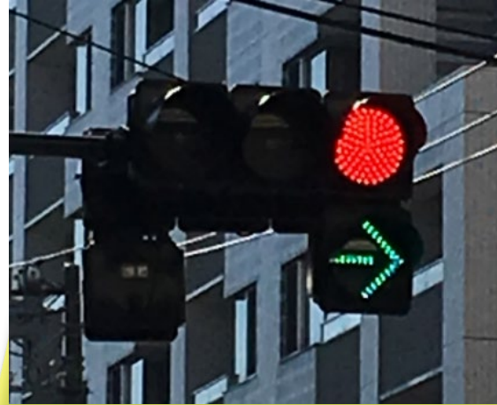
Traffic control & management
